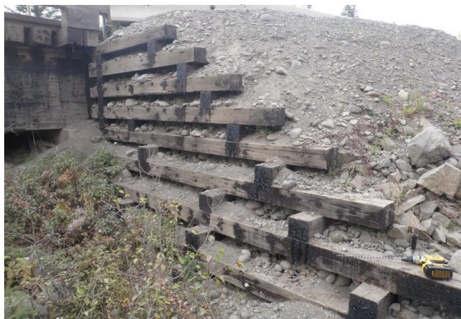
Figure 1-25: Woods end downstream wing wall.
