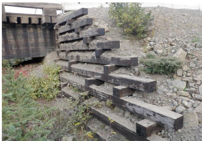
Figure 1-28: Camp end upstream wing wall.
