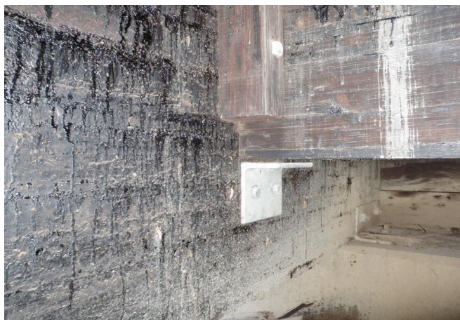
Figure 1-20: Typical downstream connection of diaphragm.
