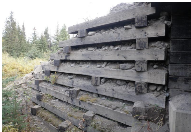
Figure 1-29: Camp end downstream wing wall.
