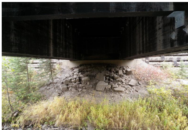
Figure 1-26: Camp end abutment.
