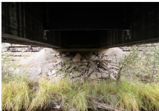
Figure 1-22: Woods end abutment.
