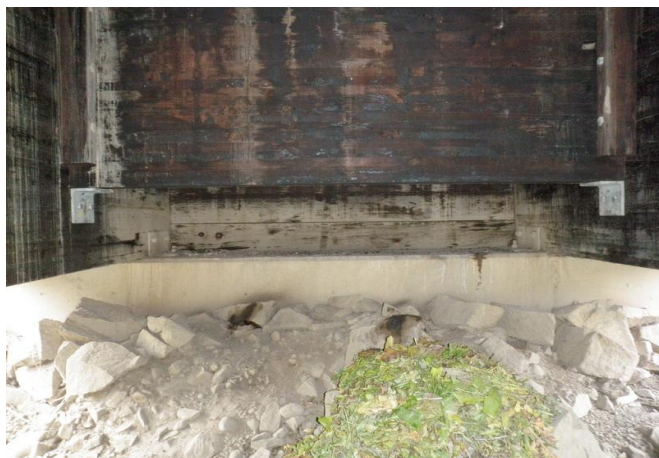
Figure 1-23: Woods end abutment.
