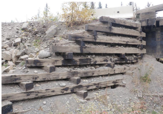
Figure 1-24: Woods end upstream wing wall.
