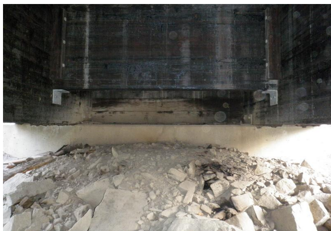
Figure 1-27: Camp end abutment.
