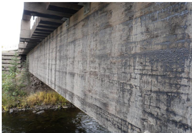
Figure 1-19: Girder 4 downstream face.
